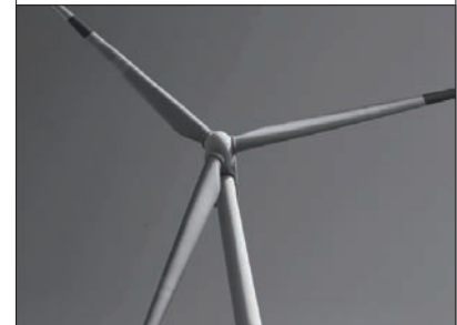
wind blade deformation inspection
